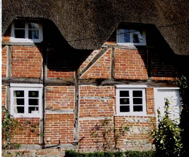
*6 & 7 Mill Lane timber frame with brick infill*
