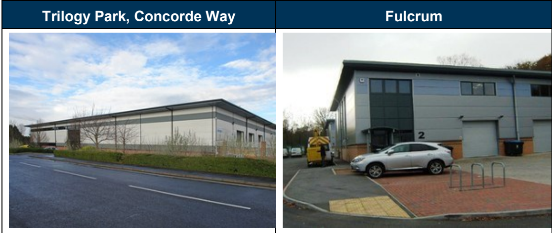
Figure 4.3 Examples of industrial units, M27 Corridor – Whiteley
